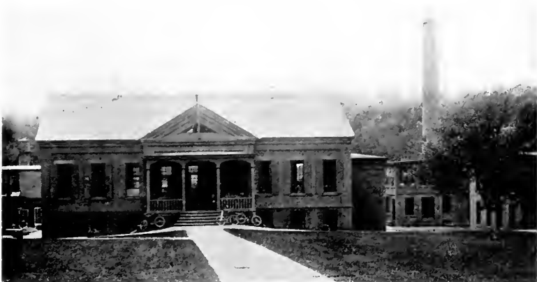
THE OFFICES AND A GLIMPSE OF THE MILLS.
